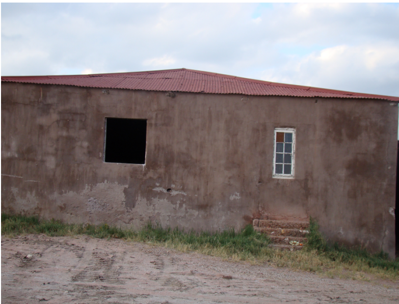
Figure 18- Historic building at the Saltpan Cave industrial site
