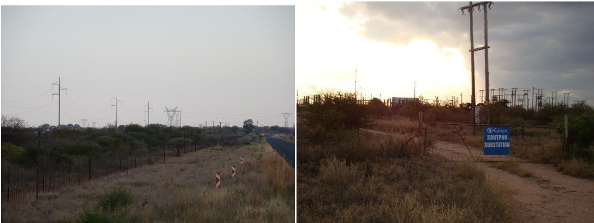
Figure 19 - High-voltage Lines leading to Saltpan Substation - Option 2
