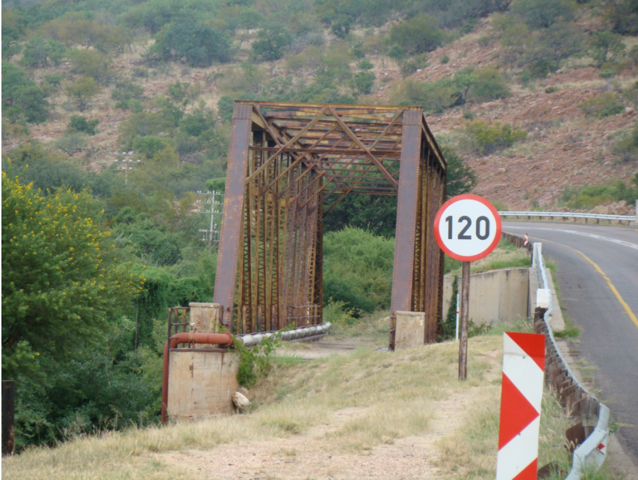
Figure 16- Historic bridge north of the Soutpansberg Mountain and some KMs south of Option 1 to Nzhelele.
